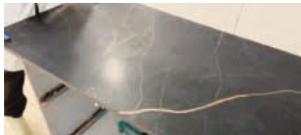
Place the porcelain slab on top of the module. Collocare la lastra sopra il mobile.
